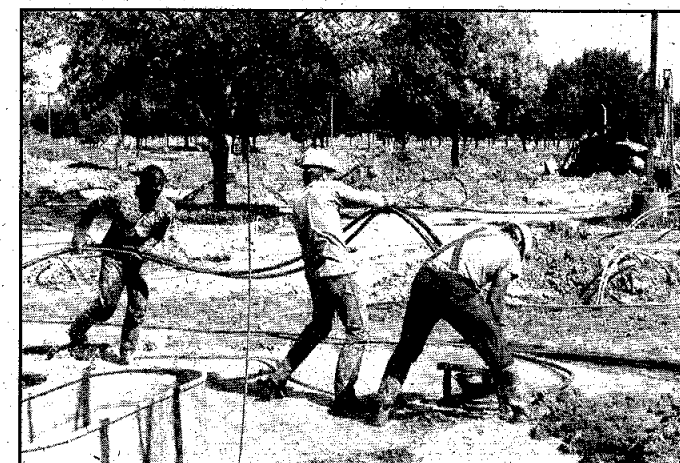
Workers push a folded length of polypipe into the borehole.
