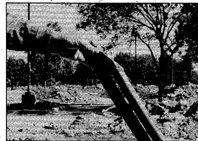
Each length of uncoil polypipe folds at a U-bend installed at the factory.
