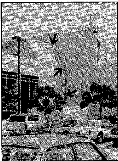
Covered riser for heat exchanger (indicated by arrows) installed at the Sun Publishing Company.
