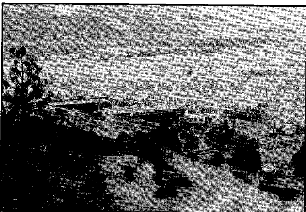
Now under operation, power plants PLES I (left) and Mammoth Pacific II (right). At first glance, they seem to be one large power plant. However, closer inspection shows the two plants are offset (center photo), with the banks of cooling towers at different levels. Steam from a fumarole wafts at photo right, front.
