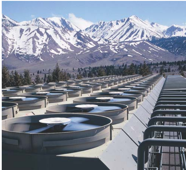
Mammoth-Pacific's fin fan condensing system relies on air cooling, but performance—and power output—suffer during the hot summer months.
