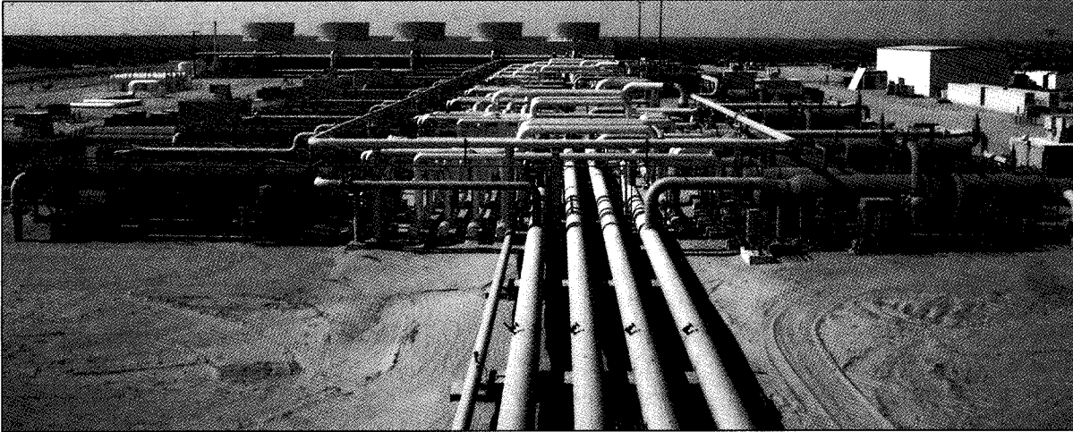
ORMESA I Power Plant comprised of 26 modular Ormat Energy Converters with 30 MW nameplate capacity, synchronized to the IID grid in December 1986.
