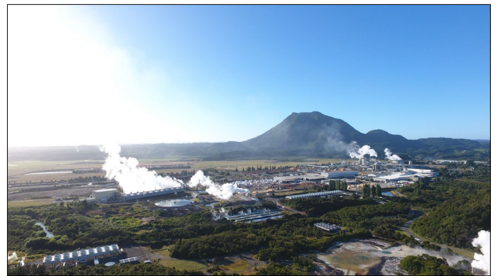
Kawerau industrial site (Courtesy Ngati Tuwharetoa Geothermal Assets)
