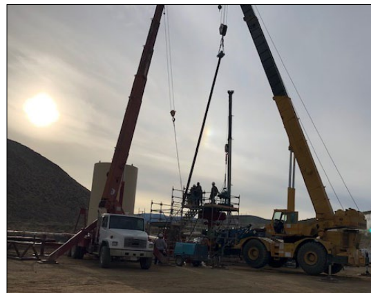
The vacuum insulated tube (VIT) is inserted into the well. Courtesy Chris Ellis
