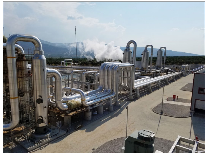
Kizildere-3 C, by Matt Fishman, POWER Engineers, Inc. 65 MW Kizildere-3 Unit 1 Geothermal Power Plant, Turkey, August 18, 2017. GRC Photo Contest 2017.
