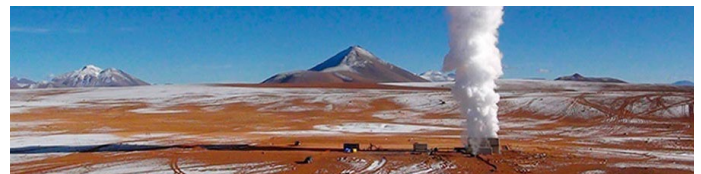
Laguna Colorada geothermal facility (Courtesy ENDE)
