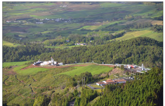
Ribeira Grande geothermal power plant on São Miguel Island in the Azores. Courtesy EDA Renováveis, S.A.
