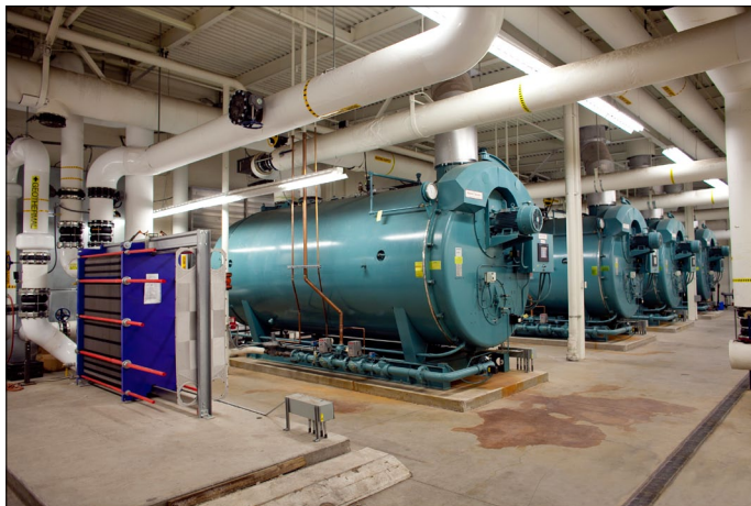
In case of a geothermal system failure, the Peppermill still has the boilers that were used before the sustainable system went online.
