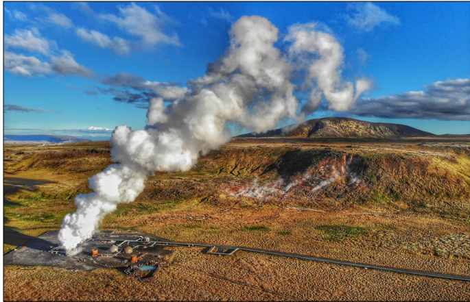
Hellisheiði geothermal power plant. Courtesy Lydur Skulason of Deilir Technical Services, Kópavogur, Iceland.
