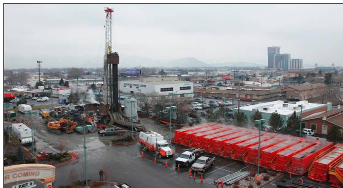
Drilling of injection well #9.
