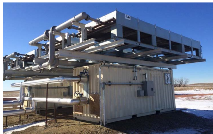
Figure 4. ORC units as installed at the Davis Water Injection site.
