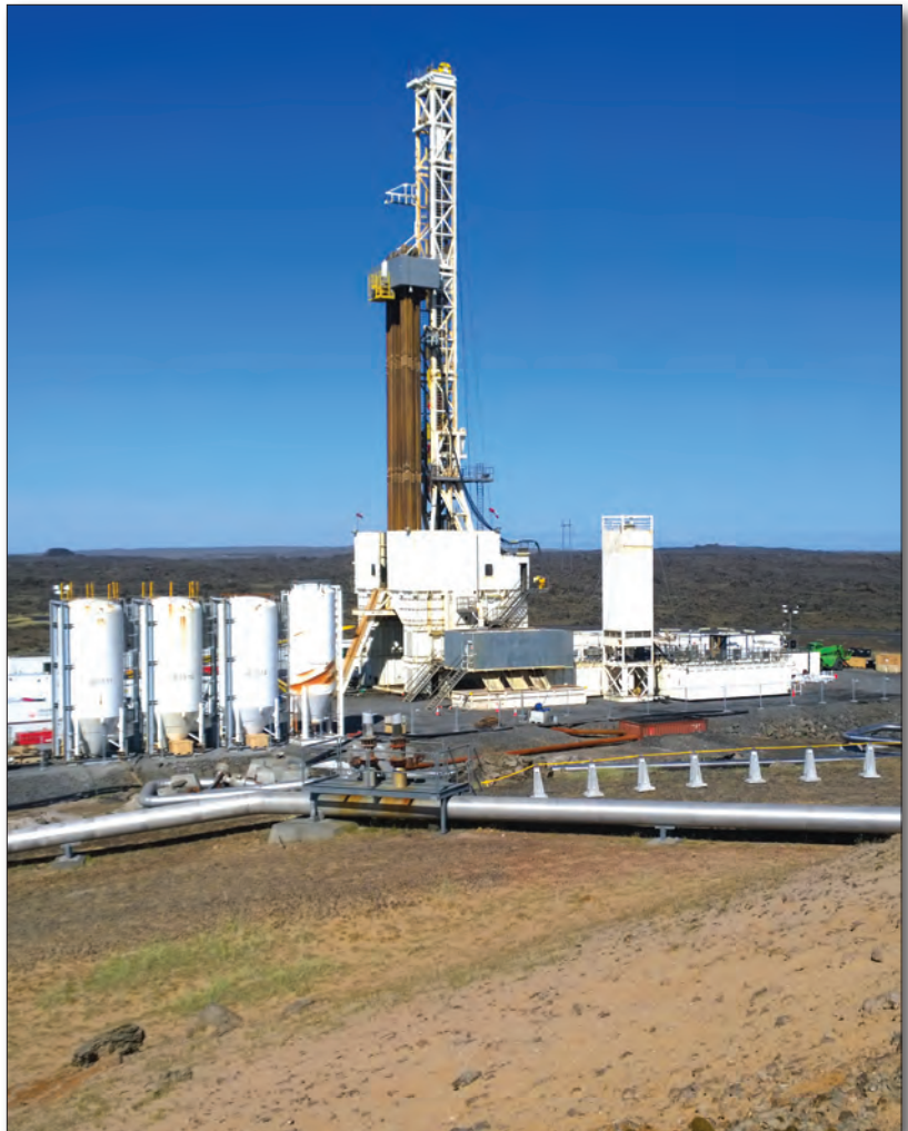
Drilling rig Thor at IDDP-2 site at Reykjanes (Guðmundur Ó. Friðleifsson)
