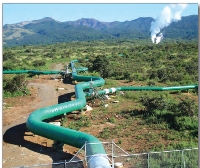
Pipeline in Las Pailas I, by Paul Moya. Two phase pipeline coming to the separation station at Las Pailas I, Costa Rica. Photo was taken in July 2011. GRC PHOTO CONTEST 2016
