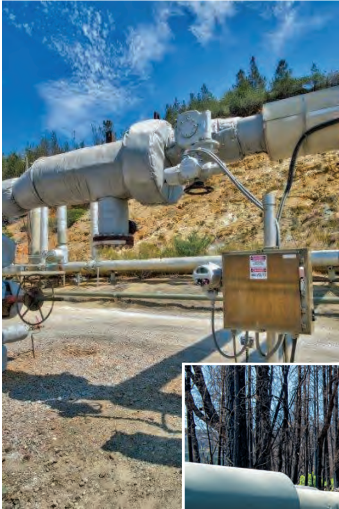
Figure 3: This new steamflow control valve actuator is designed to allow remote reduction of steamflow to plants.
