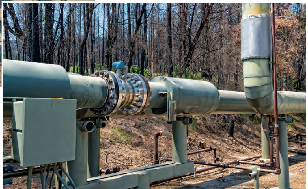
Figure 4: This vortex-shedding flow meter measures flow rates at a better turndown ratio than an orifice plate. It is currently being evaluated to determine its turndown accuracy.
