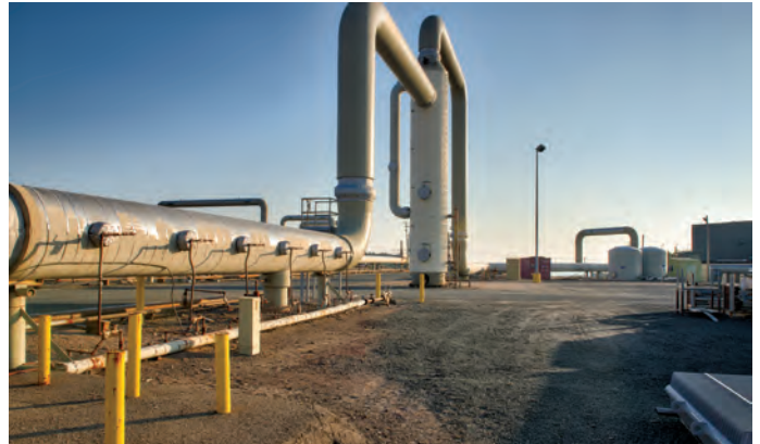
Figure 5: Injecting condensate upstream of a separator to scrub chlorides.
