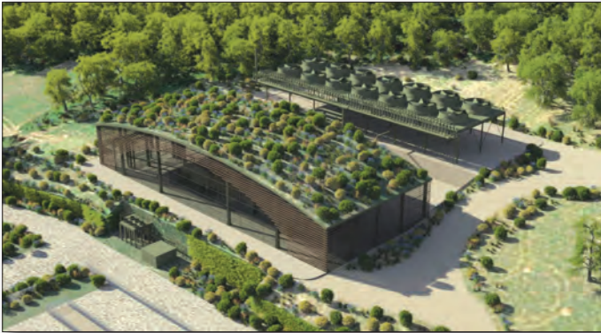
Spot the power plant! Artist rendering of the next-generation geothermal power station being built by GGP in the Val di Cecina region of Italy. COURTESY GE OIL AND GAS
