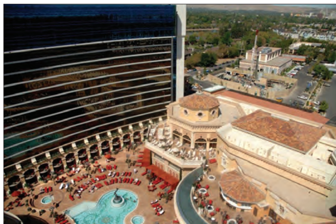
The Peppermill pools with the #8 Production Well being drilled in 2009 in front of the Central Plant facility. COURTESY PEPPERMILL
