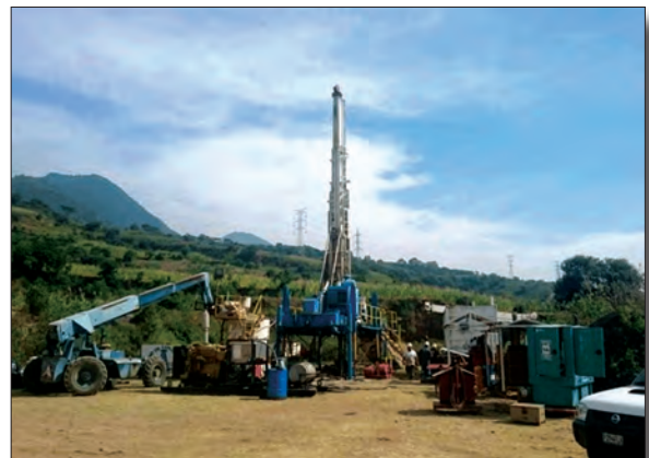
Drilling on EC-2 at El Ceibillo. COURTESY U.S. GEOTHERMAL INC.
