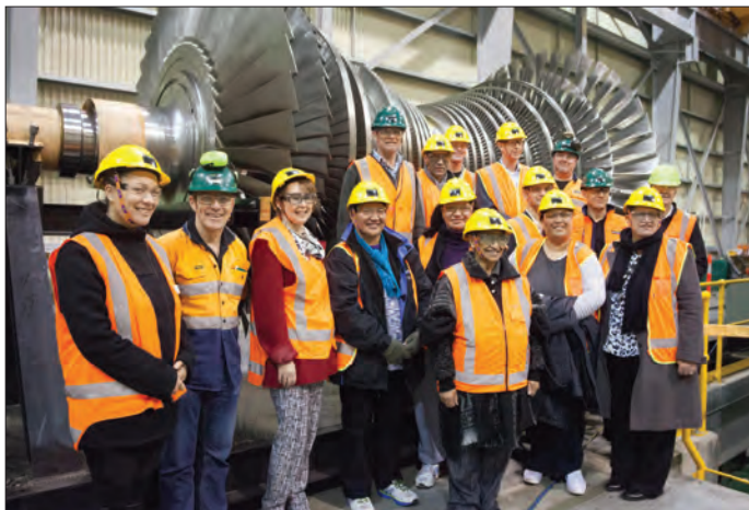
Everyone is happy to see a new turbine installed. COURTESY MIGHTY RIVER POWER
