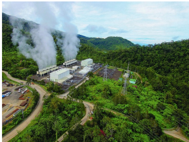
Figure 4: Mindanao I and Mindanao II geothermal power plants
