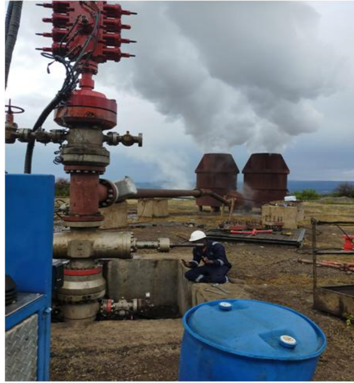
Figure 13: MW-08 discharging during air-lifting
