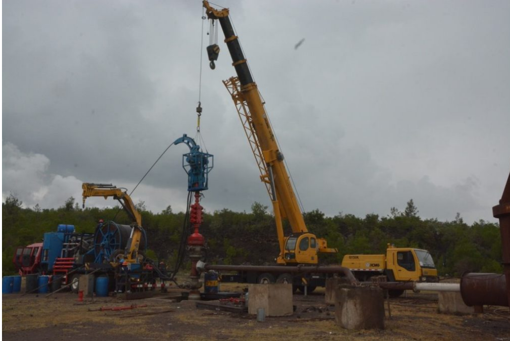
Figure 5: Coiled tubing assembled on the well head
