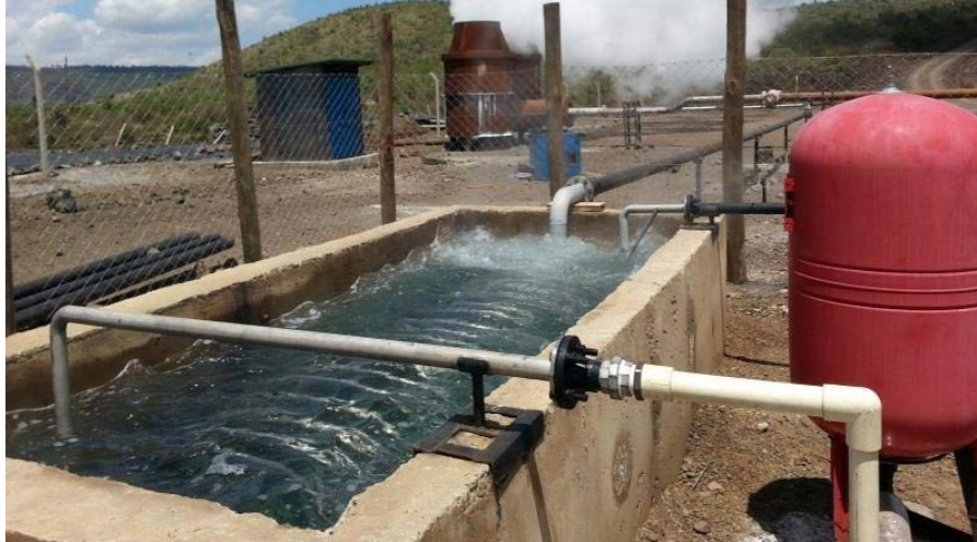
Figure 7: Heat exchanger at well MW_03
