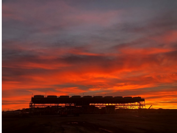
Figure 6: Lightning Dock geothermal power plant
