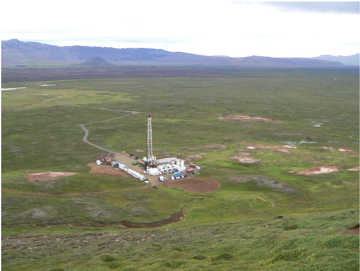
Figure 6: Exploration drilling with the rig Jötunn at Theistareykir area 2006 (Thg-3).
