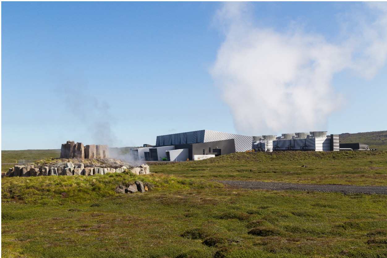
Figure 10: Theistareykir Geothermal Power Plant in full operation
