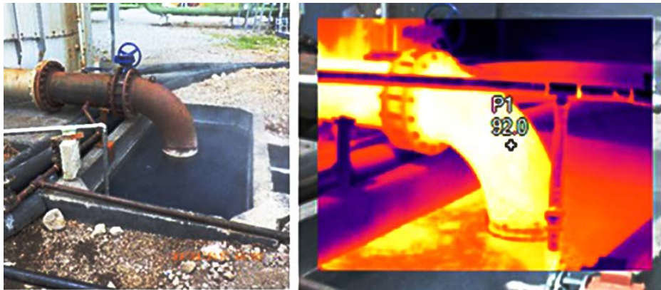
Figure 5 Geothermal fluid dump and temperature measurement with a thermographic camera.
