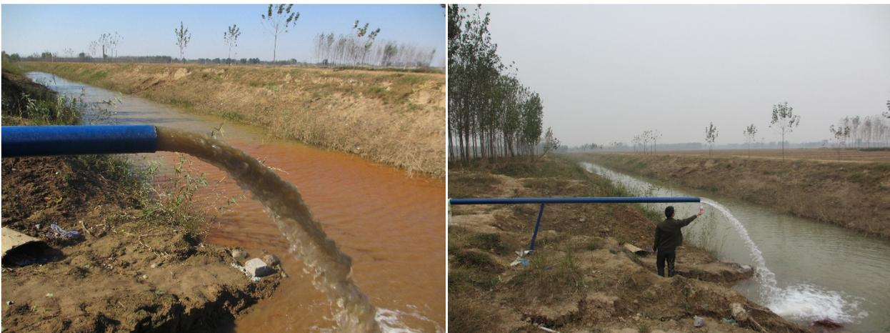
Figure 11: Re-pumping during the reinjection until the re-pumped water to be clear and without sand (Left-at the beginning of re-pumping; Right-at the end of re-pumping)
