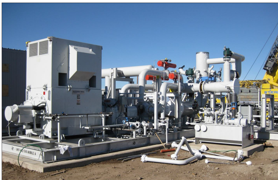
Figure 8. Photograph of the Paisley Power Plant generator, turbine, heat exchanger, and condenser piping.
