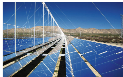
(c) linear Fresnel reflectors
