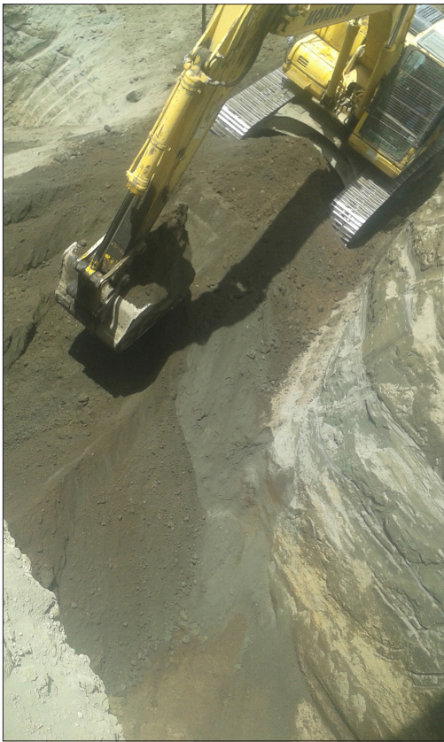
Figure 2. Civil excavations works.
