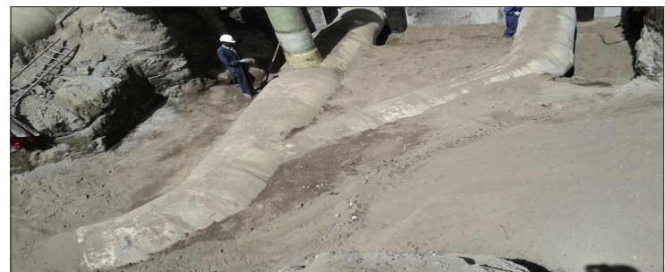
Figure 4. Construction in Progress. Glass Reinforced Plastics pipe installations.
