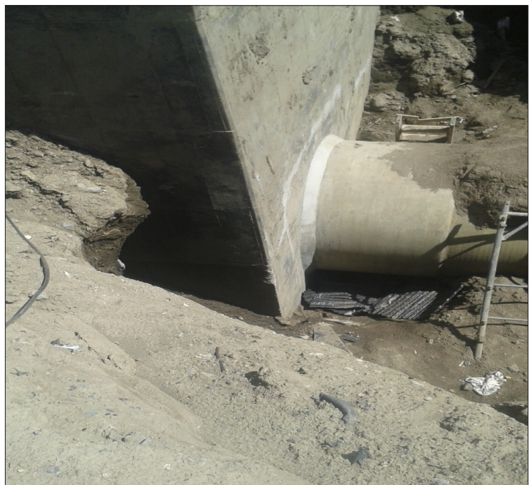
Figure 5. GRP pipe at the connection of the hot well area.
