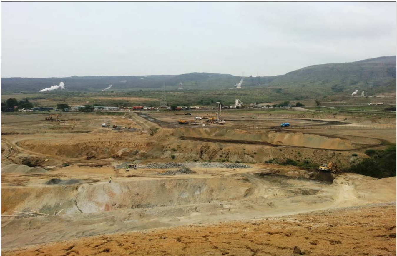
Figure 7. Initial stages of project construction.-Site clearance and earthworks.
