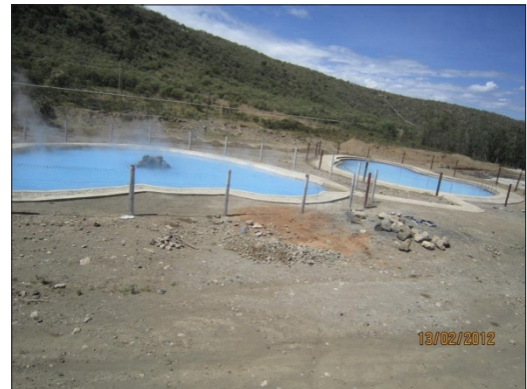
Figure 6. The spa during construction...Landscaping.
