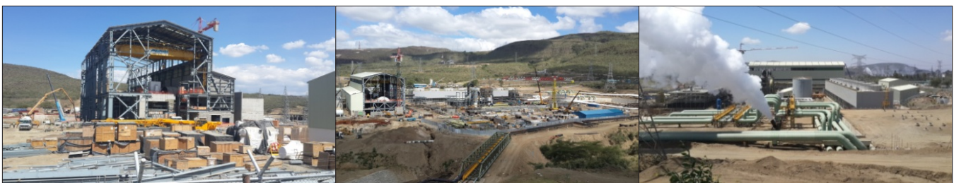
Figure 8. The plant during construction.
