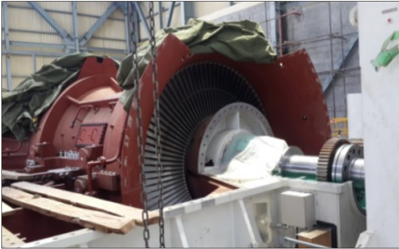
Figure 9. Turbine during installation.
