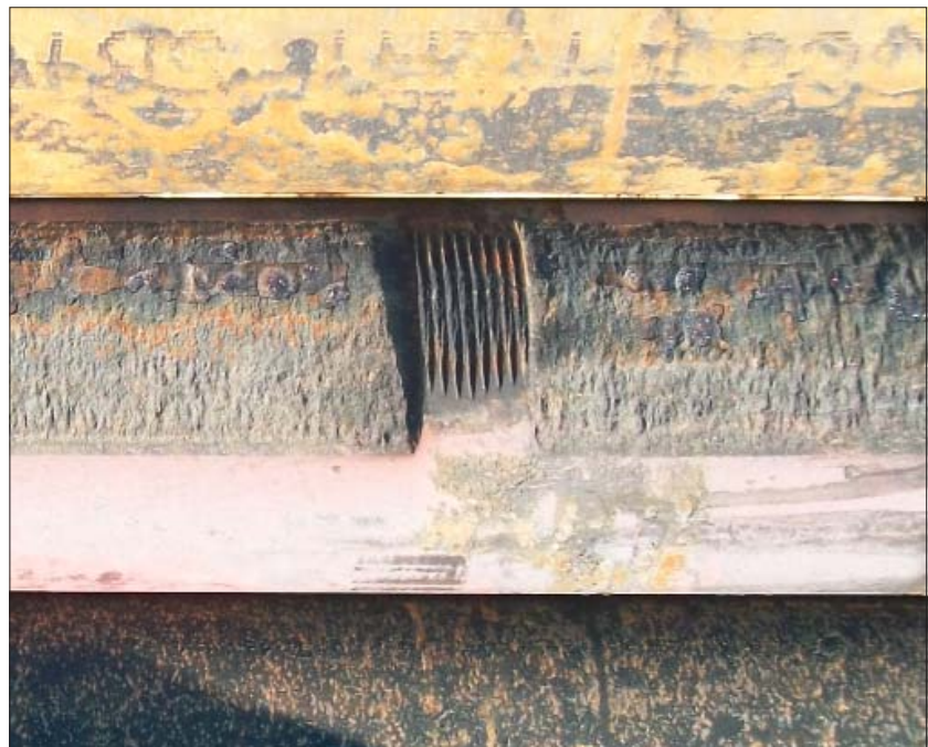
Figure 8. Signs of column contact on lineshaft enclosing tube.
