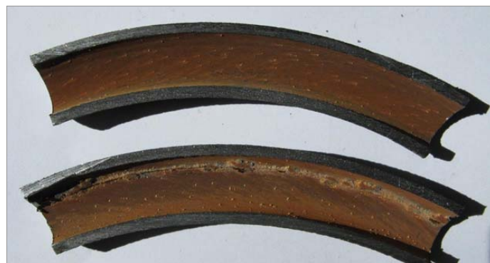
Figure 6. Sample 14 (untreated position 4) pipe section.
