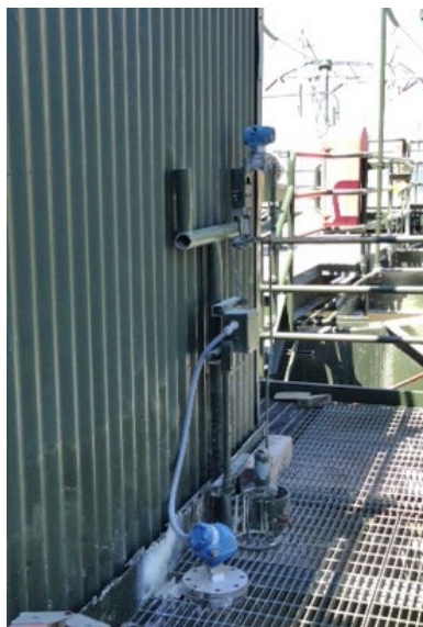
Figure 3. Unit 18 Balance Tank Non-Contacting Radar Installation.
