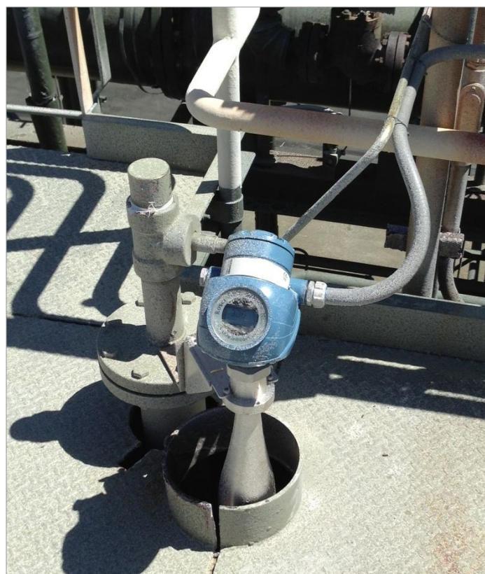
Figure 4. Unit 18 Froth Tank Non-Contacting Radar Installation.
