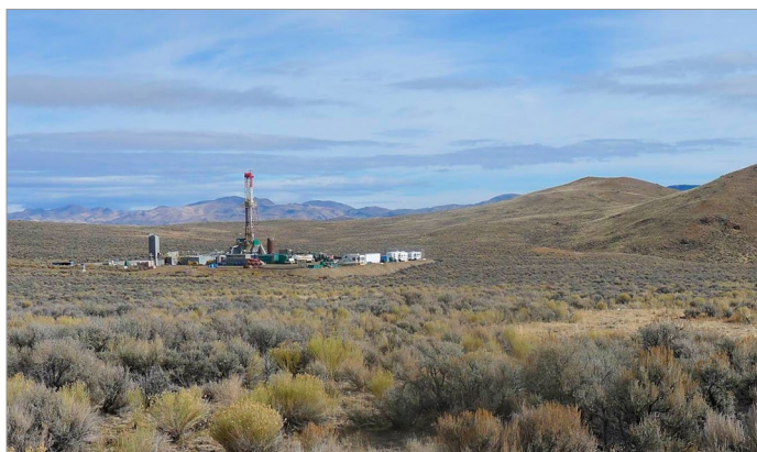
Figure 3. Well drilling at the McGinness Hills project.
