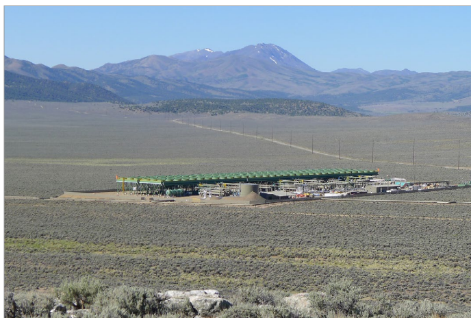
Figure 10. The completed McGinness Hills power plant.
