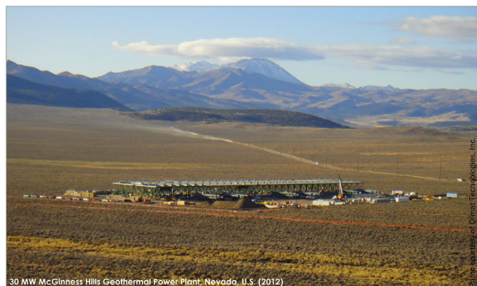
Figure 9. The McGinness Hills power plant under construction, 2012.
