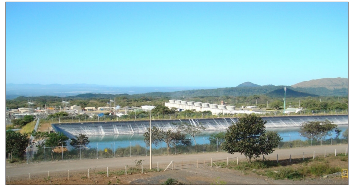
Figure 10. Overview of plant, looking generally west; holding pond for cold reinjection in foreground; the main road is off to the right, roughly parallel to the cooling tower. Photo by P. Moya.
