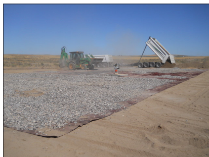
Figure 4. Kimama site preparation.
