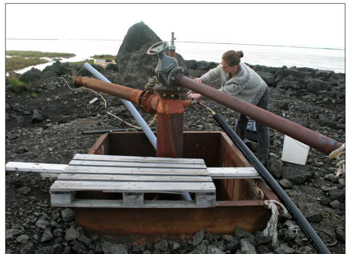
Figure 2. At wellhead of BA-04 in Keldunes. The Jökulsá river is seen in the background.
