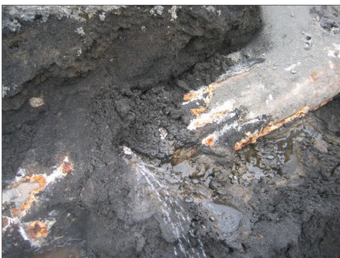
Figure 8. Tension cracks with water seeping out.
