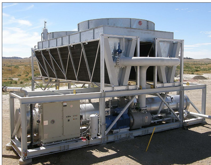
Figure 1. The RMOTC OEC, commissioned in September 2008.
