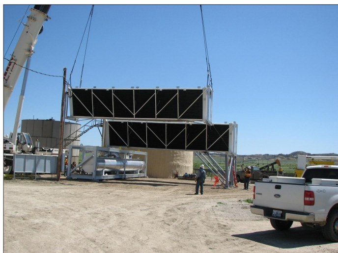
Figure 4. The OEC was installed and commissioned in approximately 4 weeks.
