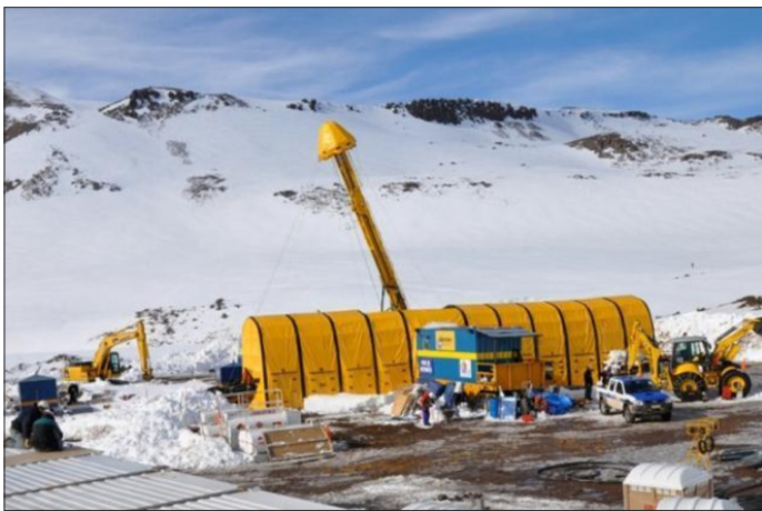
Figure 7. Slimhole MP 03 drilled under winter conditions where seasonal snow fall exceeded 5 m.
