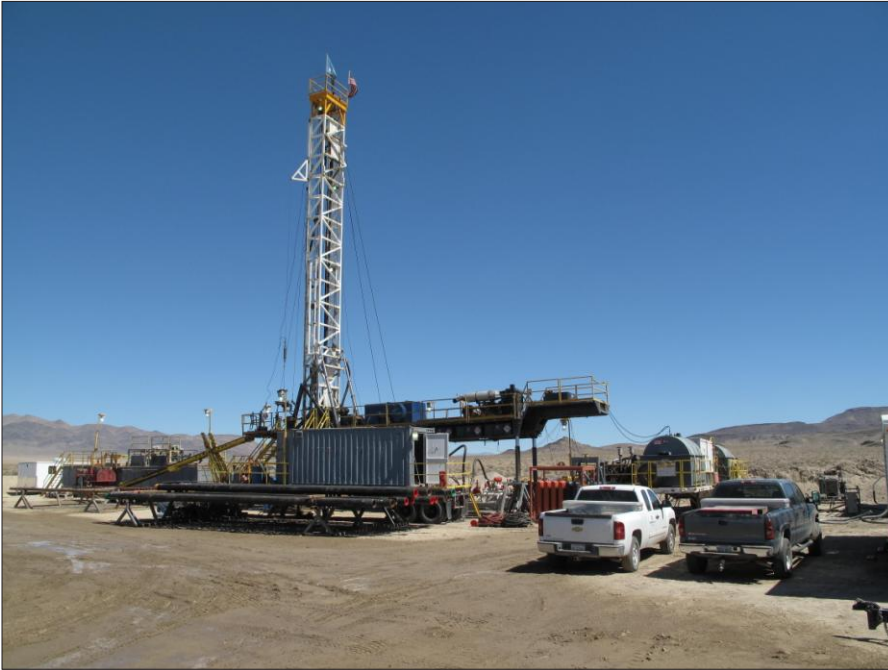
Figure 2. Drill Rig 77 on site at HAD-1, Hawthorne Army Depot, Hawthorne NV.
