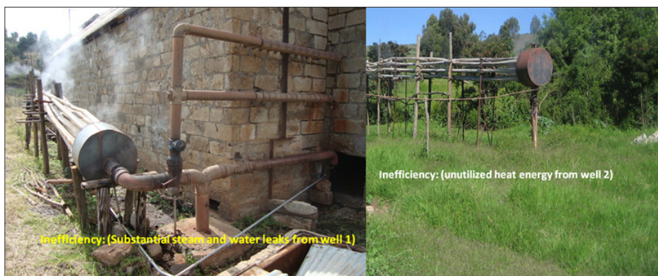
Figure 4. Inefficient Utilisation of the geothermal energy.
