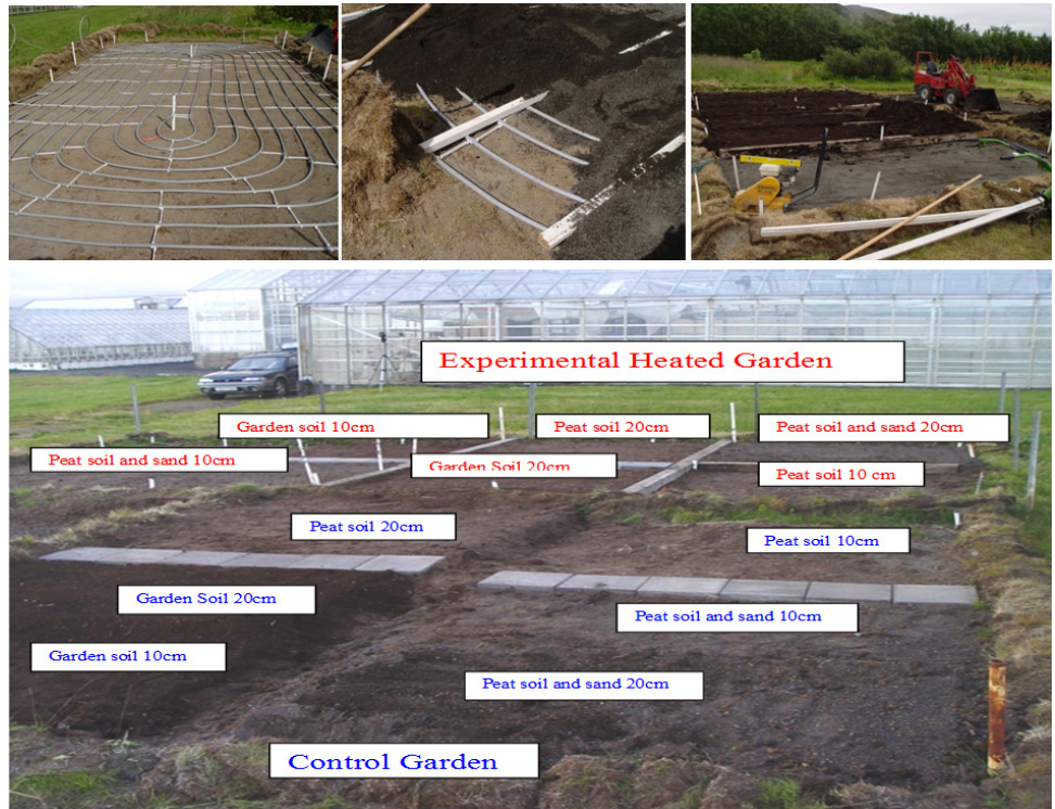
Figure 2. Hveragerdi spiral piping layout (top left), sand over layer construction detail (top center), soil top layer and gravel compaction construction detail (top right), soil depths, types and location (Bottom).
