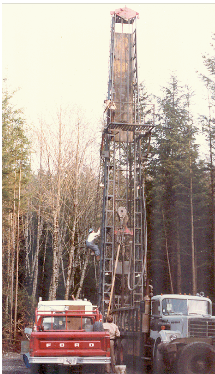
Figure 3. Photo of temperature gradient drilling in the Black Diamond area (Vice, 2010).
