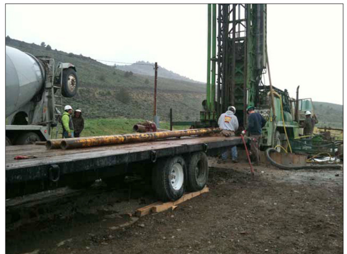
Figure 3. Paisley Drilling May 2011.
