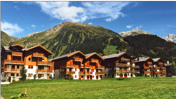
Figure 3. Oberwald/VS – a distributor network at the western portal of the Furka Rail Tunnel conducts the tunnel water to the heat pumps for each consumer. Tunnel water temperature: 16° C, thermal capacity: 960 kW (Photo: J. Wilhelm, Pully).
