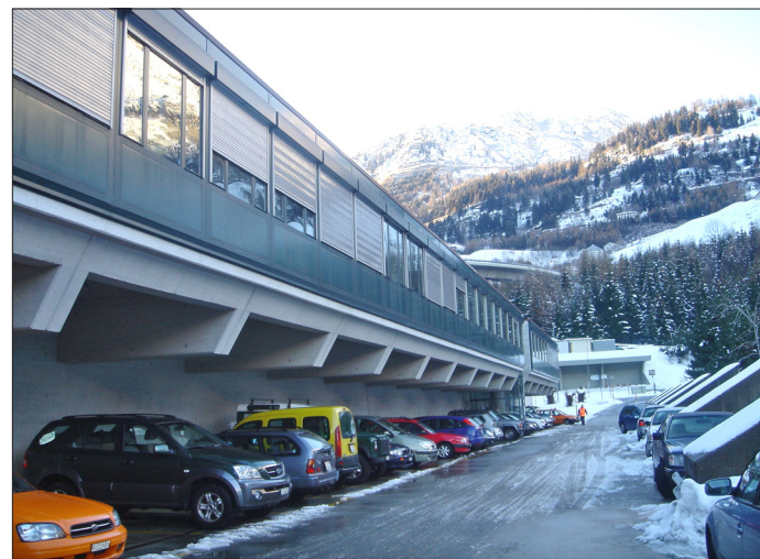
Figure 2. Airolo/TI – The Services Centre of the Gotthard Road Tunnel at the southern portal has been heated and cooled geothermally since 1979. Tunnel water temperature: 17° C, thermal capacity with 4 heat pumps: 720 kW (Photo: Geowatt AG, Zurich).
