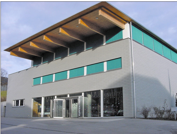
Figure 4. Kaltbrunn/SG – a multipurpose building, a gymnasium, a civil defence facility and a kindergarten are heated with the help of a heat pump at the southern portal of the Ricken Rail Tunnel. Tunnel water temperature: 12° C, thermal capacity with 2 heat pumps: 156 kW (Photo: www.geothermie.ch ).
