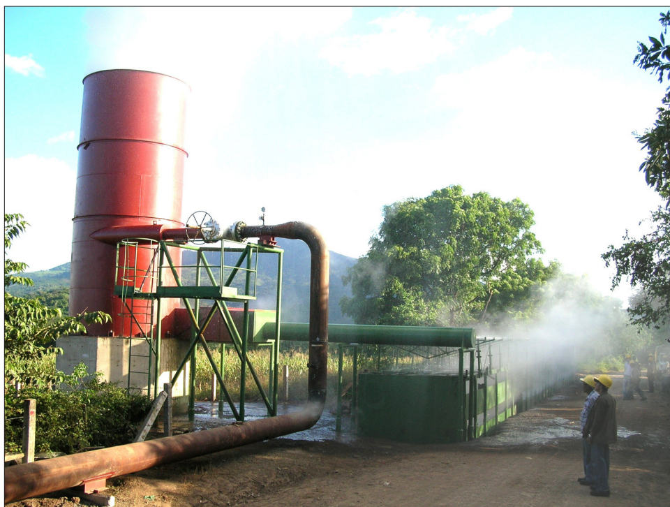
Figure 1. Flash tank and improvised cooling system for cold brine injection.
