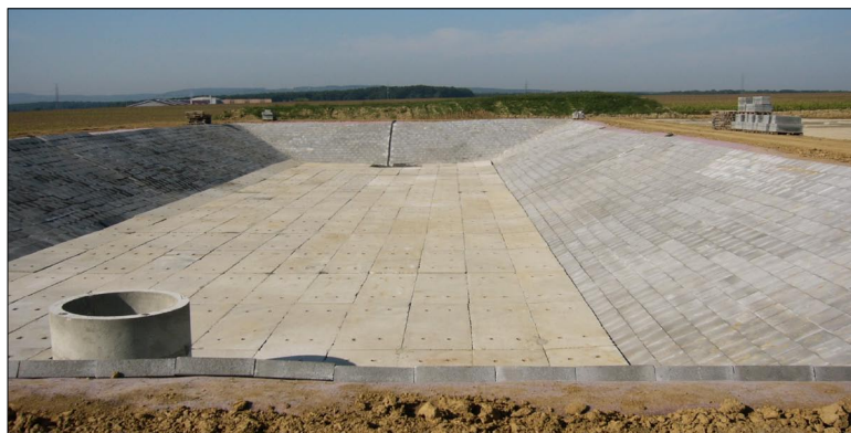
Figure 3. Construction of a 2000 m 3 pit for well testing.
