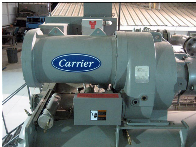
Figure 2. Chena ORC1 turbine/generator assembly analogous to Carrier motor/compressor assembly.
