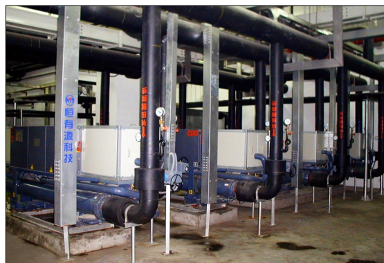
Figure 2. Building Mechanical Room.
