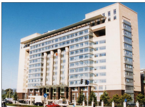
Figure 1. Beijing Haidian District Government Office Building.
