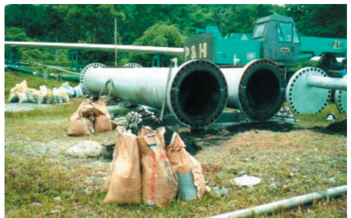
Figure 11. Solids debris collected from the MST.
