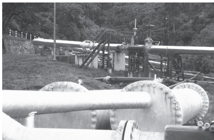
Figure 3. The new modified solid trap at 1R8D.
