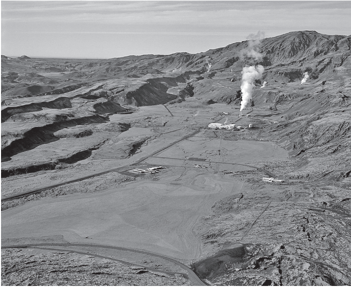
Figure 2. Existing geothermal power plant at Nesjavellir, operational in 1990.
