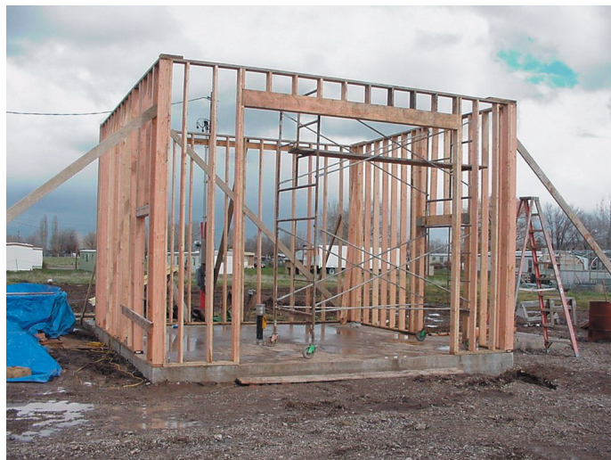
Figure 2. Beginnings of the I'SOT geothermal district heating central plant, May 5, 2003.
