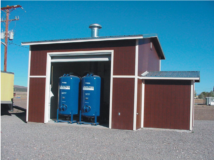
Figure 3. Completed central plant with granulated activated carbon (GAC) vessels.
