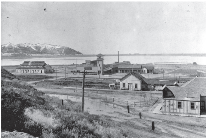
Figure 2. Two historic photographs: the Warm Sulfur Springs Bath House, completed November 27, 1850 (top); and Beck's Hot Spring resort sometime before 1898 (bottom). At first, mule trains brought Salt Lake City residents without indoor plumbing to the bath house for washing and recreation. Later, trains of the Great Salt Lake and Hot Springs Railway Company brought Salt Lake visitors to Beck's.
