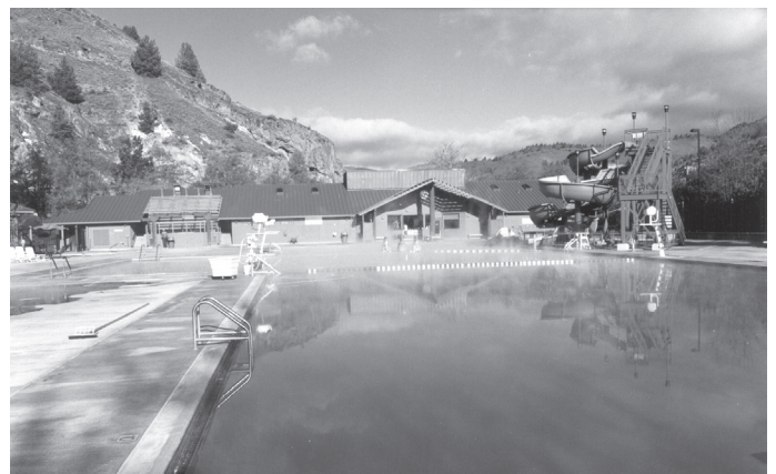
Figure 6. Outdoor pool with the slide.
