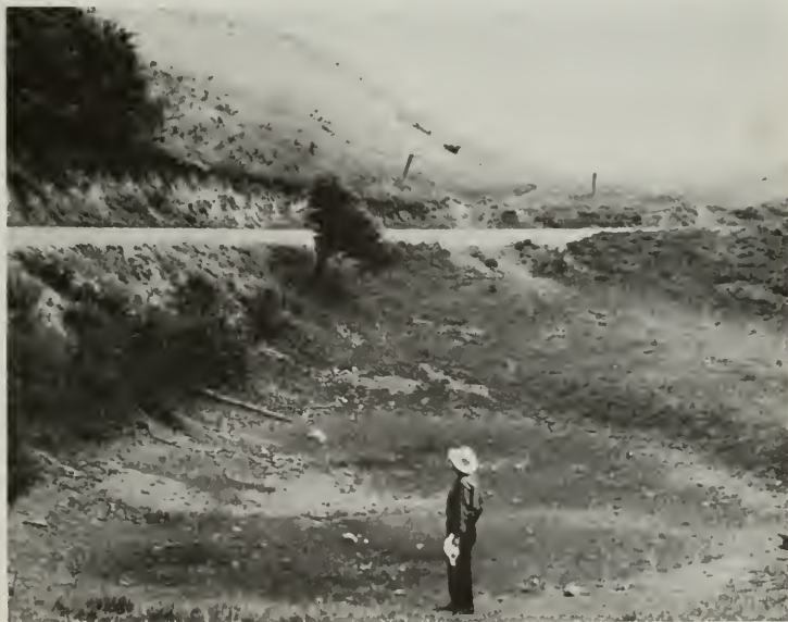
Photo 3. Sag pond and notched ridge in zone of 1906 fault ruptures at Shelter Cove, photographed looking south in 1963. Photo by K. V. Steinbrugge.
