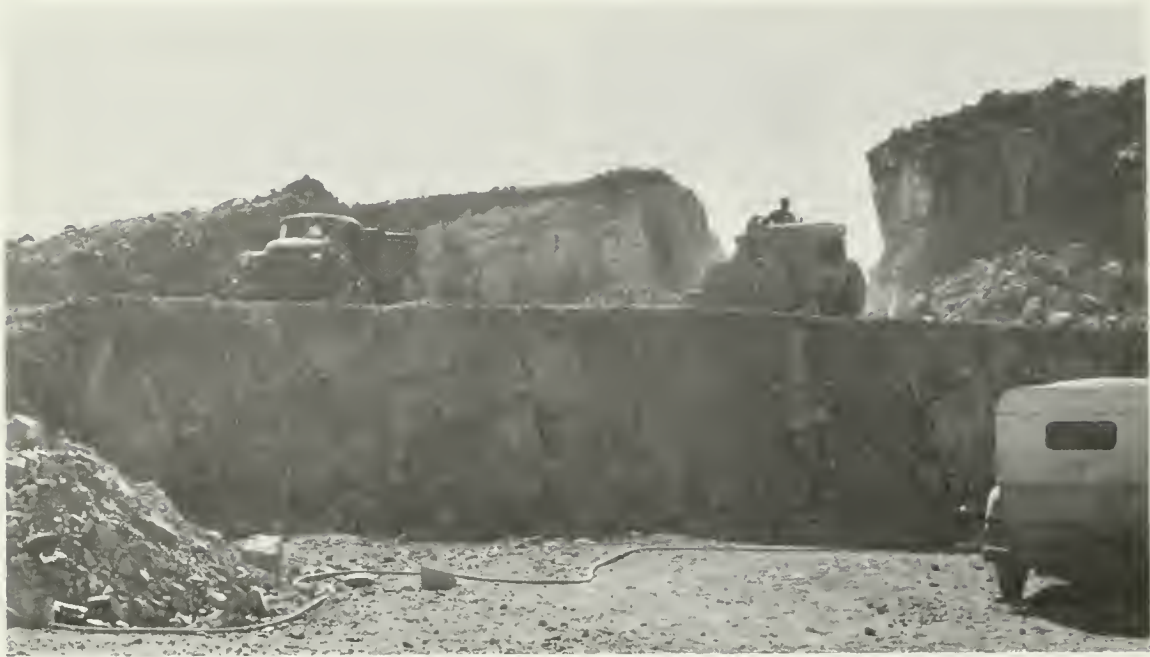
Photo 6. South Quarry, Lakeview Quartzite deposit, in March 1957: View of the northwest end of the south quarry showing initial operations in the top central part of the Eureka Quartzite. The lower face has been drilled with horizontal holes and loaded ready for blasting. The equipment on the upper bench is being used to clean up loose rock preparatory to drilling.
