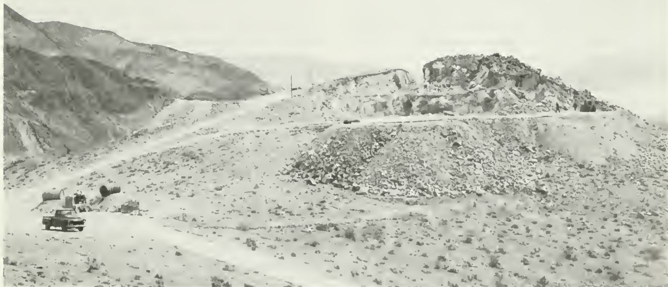
Photo 5. South Quarry, Lakeview Quartzite deposit, in 1957: View of the northwest end of the south quarry showing an early stage in the quarrying of the massive, high-purity, hanging wall beds of the Eureka Quartzite. Photo by L. A. Wright.
