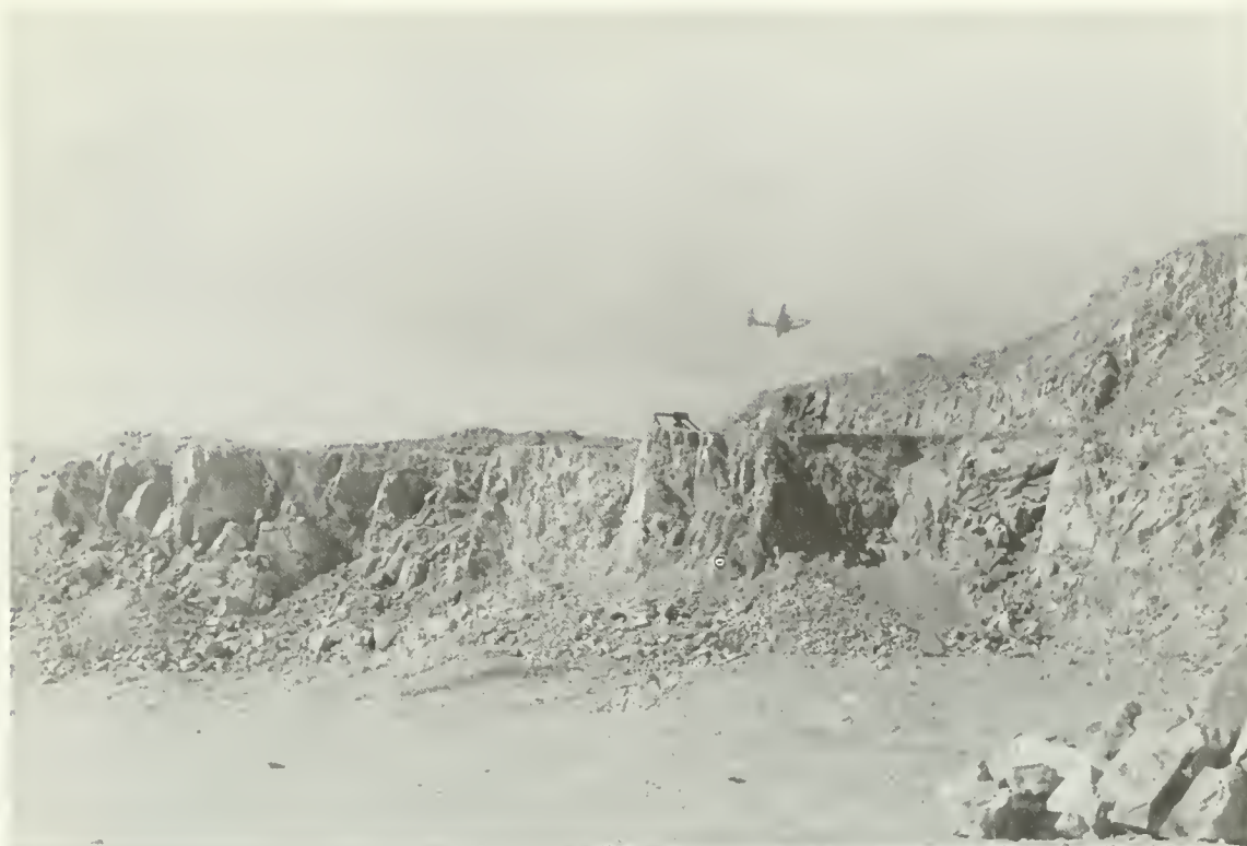
Photo 8. Atlas quarry, Mineral Materials Company: View northwest across lower bench. Since 1939, Mineral Materials Company has quarried 150,000–200,000 tons of quartzite, mostly for portland cement.
