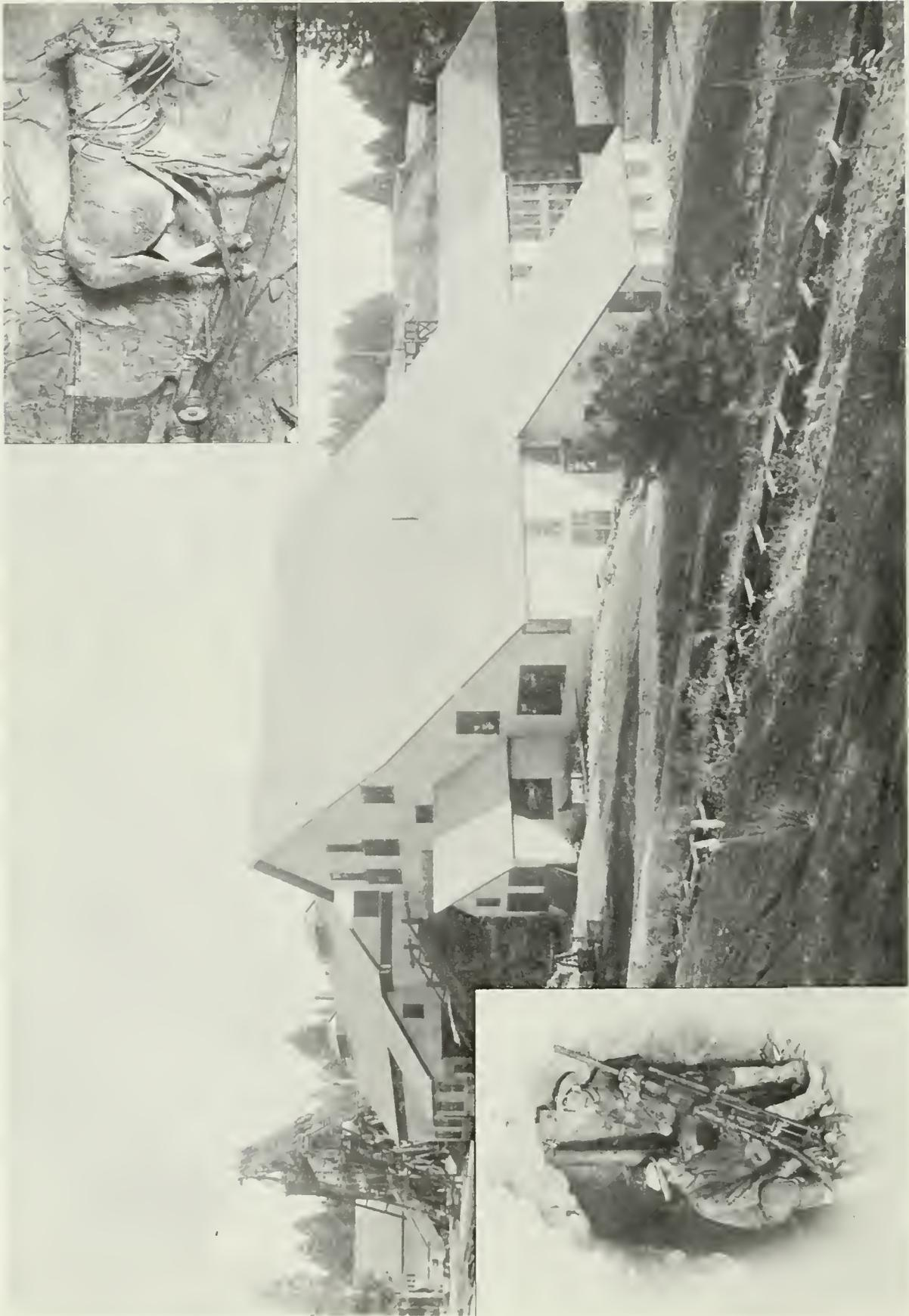
Phata 5. General view of the surface plant of the Empire Mines (lode gold), Gross Valley. Underground views (inset) show oir drilling on the 2,200 level (below) and onmal-drown ore train (above). Untavable economic conditions during ond after World War II put on end ta large-scale mining at such mommoth gold producers.
