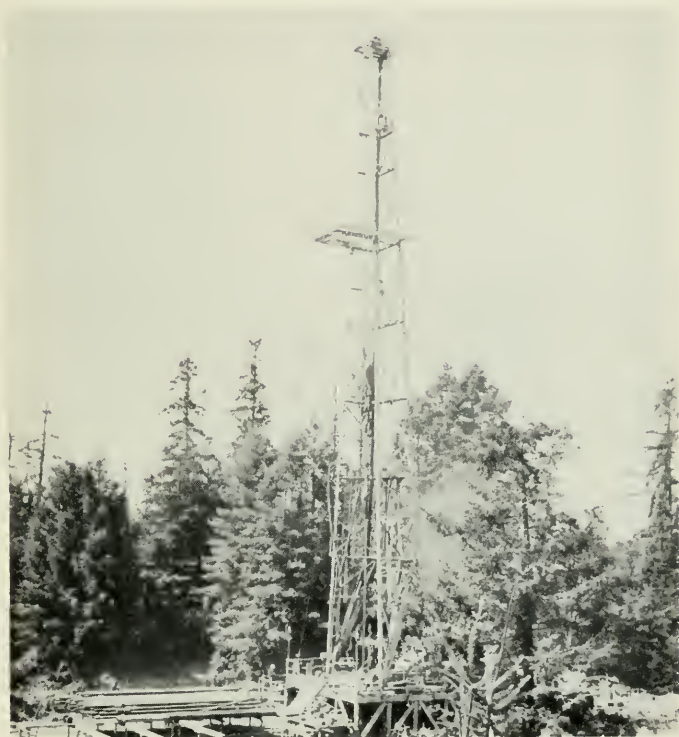
FIGURE 13. Salmon Creek Oil & Gas Co. "Fowler" 1, drilled in 1948 in sec. 15, T. 3 N., R. 1 W., H. Some oil and gas reported, but the well was abandoned.
